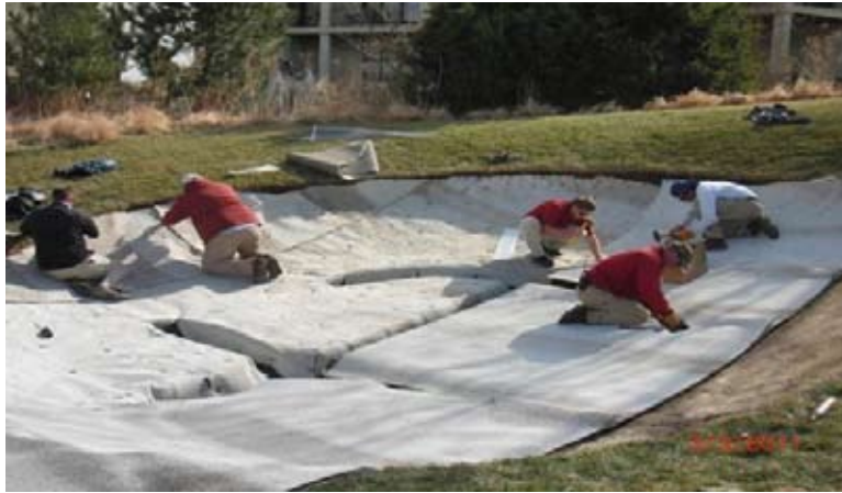
#2 left fairway bunker renovation in progress
