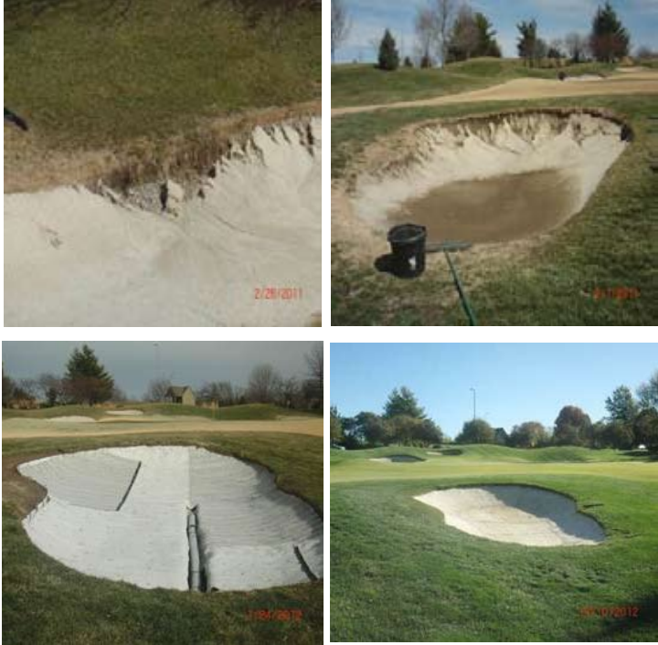
Washouts lead to contamination which leads to slow draining bunkers which increases labor costs.
