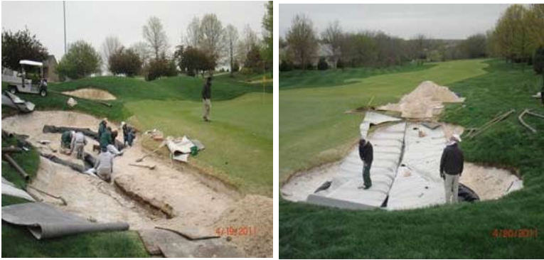
Drain liner and bunker liner installed in #6 greenside bunker
