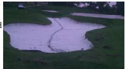
Newly lined bunker
